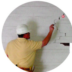
Construction supervisors and inspectors
