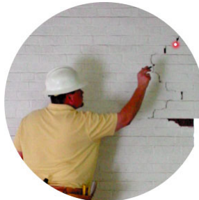
Construction supervisors and inspectors
